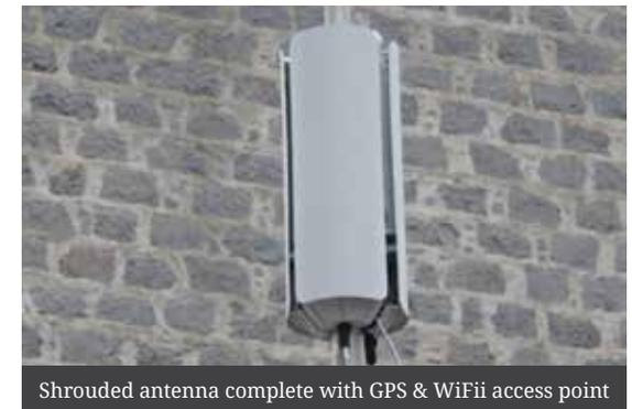
Shrouded antenna complete with GPS & WiFi access point
